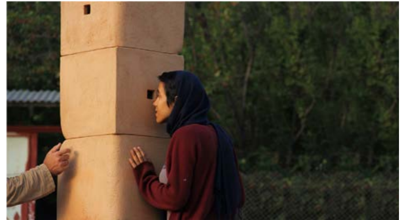
Figure 6: The second kiln-sculpture project in Polour, Iran. In the design of this kiln-sculpture, particular attention was given to the spacious interior of the structure, as well as the incorporation of openings inspired by bird nests. Photo by Reza Pourhoseini, 2015 (Author)
